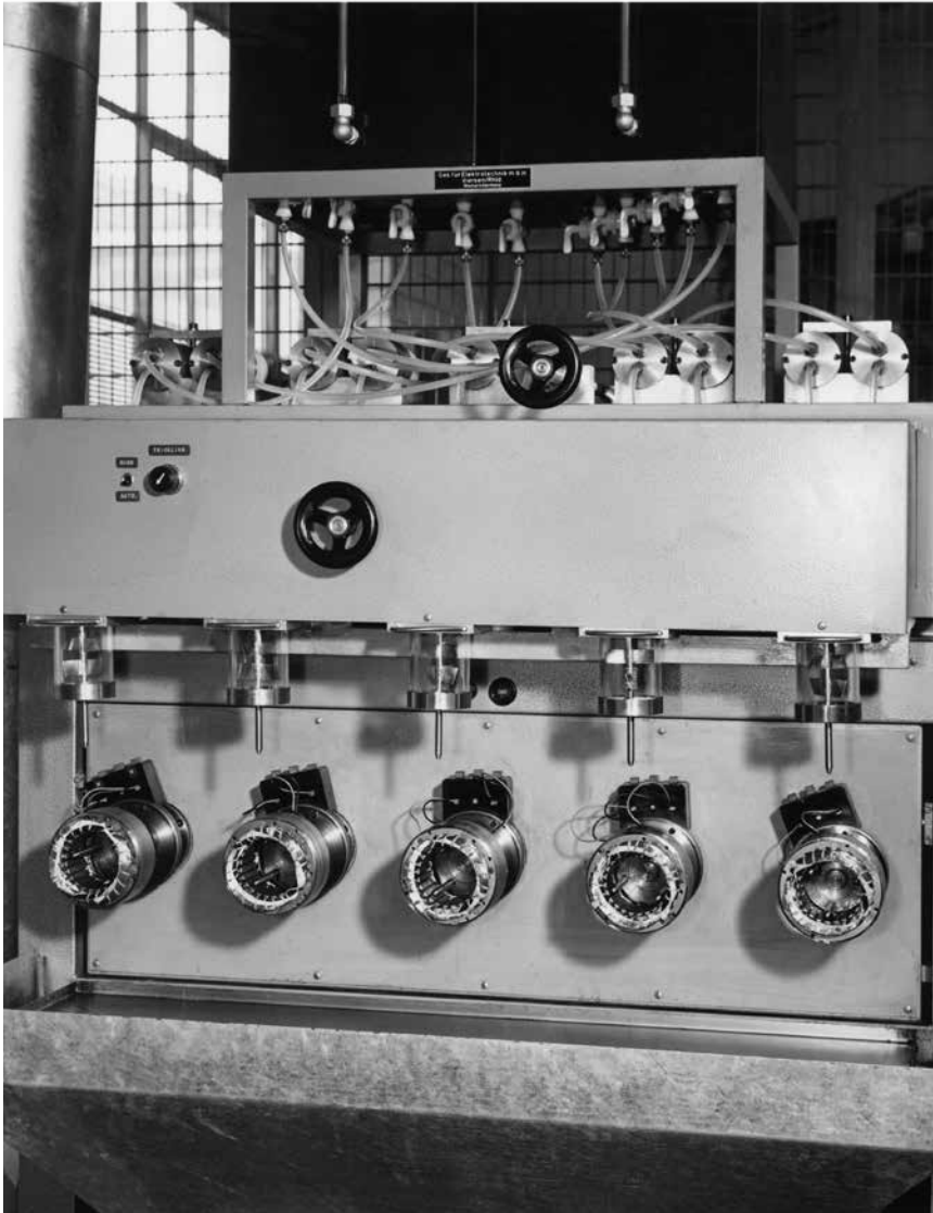
Solidly built machines: An automatic stator impregnation plant from the old times.
